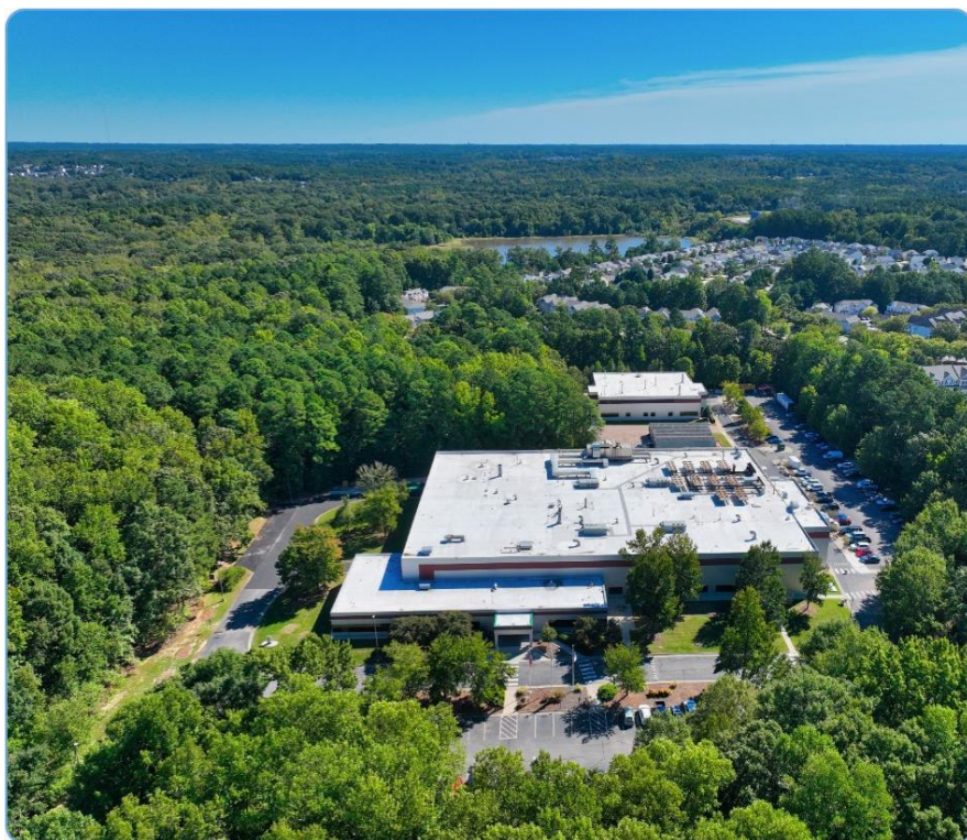
Raleigh, North Carolina facility
